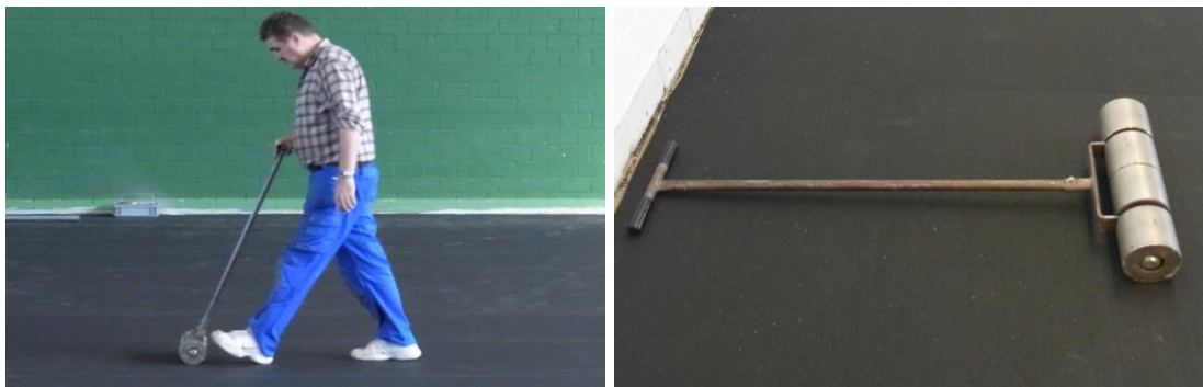
Scrolling of the floor with a pressure roller
