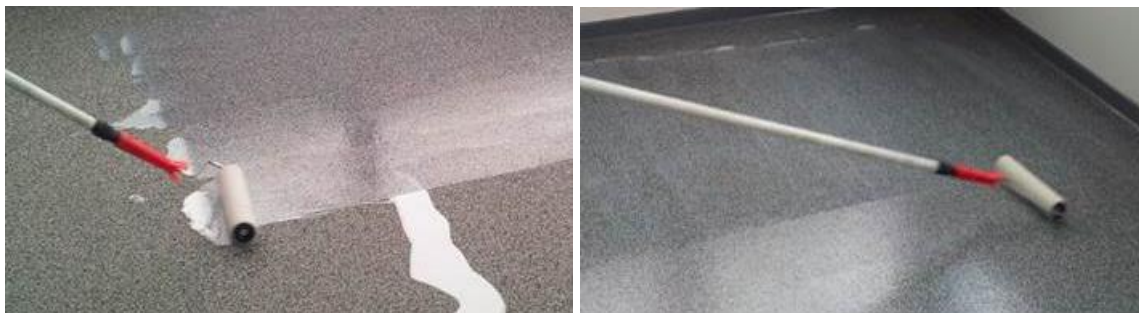
Applying of the coating
