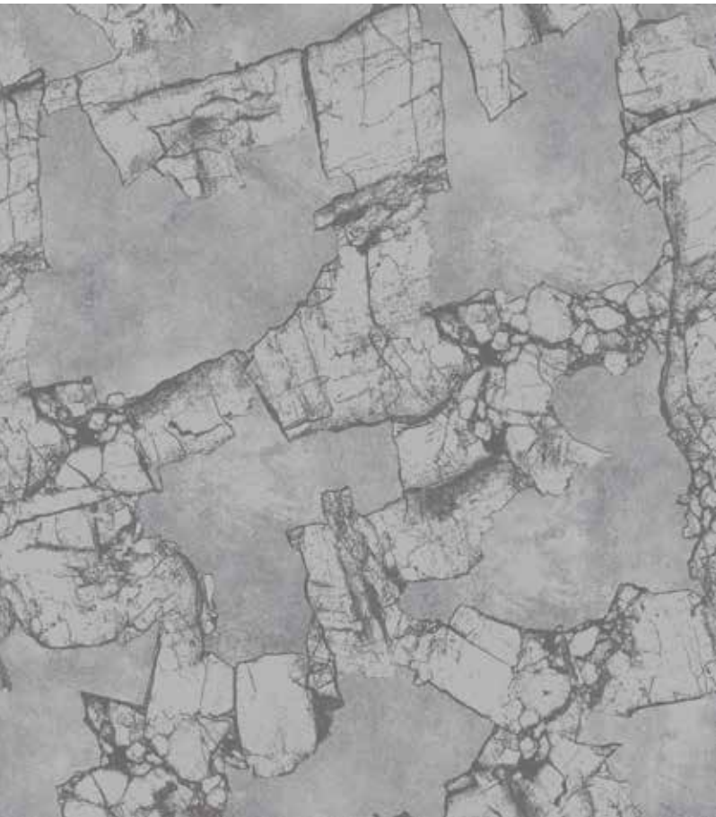
CONCRETO 90 ↔ ca. 99 X ↓ ca. 217 CM
