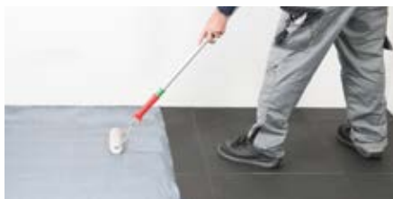
INSTALLATION WITH TACKIFIER
