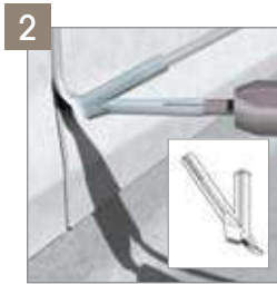
Perfect CR 41 wall weld - H231
