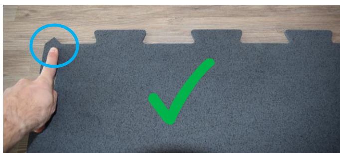
Alignment of the puzzle mat: bring the mat into position by turning or flipping
