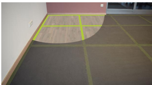
at 6mm : gluing at the edge area and at the interlocking area
